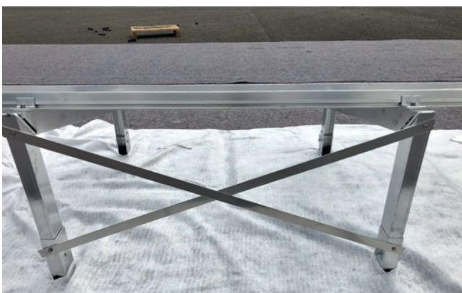
Figure 31: Wind bracing.
