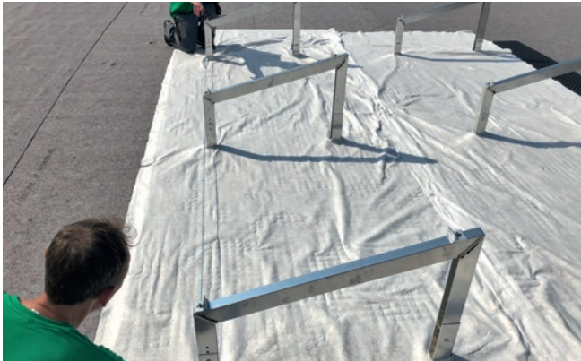
Figure 21: Alignment of the row using string
