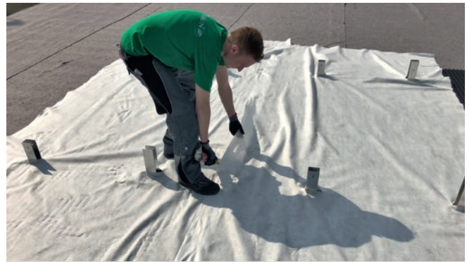
Figure 17: Bond rows of fleece with hand soldering iron
