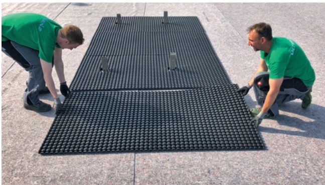
Figure 3: Installation of additional FKD 25 without Base Plate to create the spacing according to the installation plan.
