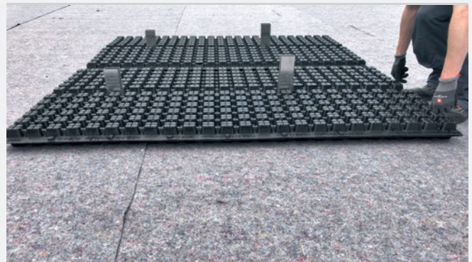
Figure 8: WRB 80FMA 8 cm with Base Plate.
