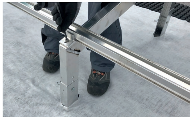
Figure 24: Tighten Rail Fixings.
