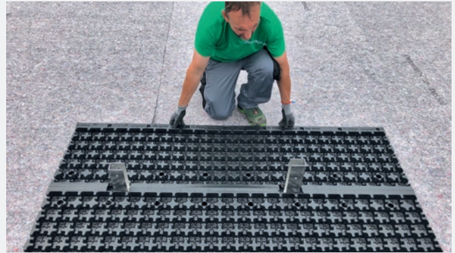
Figure 6: First WRB 80FMA placed unfolded on Base Plate.
