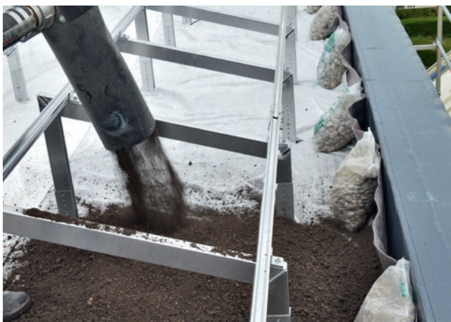
Figure 33: Blowing of the substrate.
