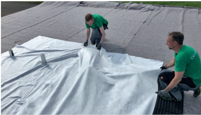
Figure 16: Lay second row of fleece.
