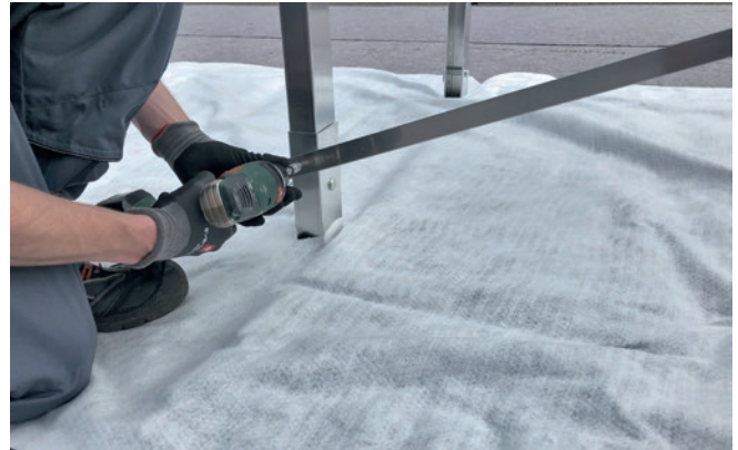
Figure 28: Fastening of the metal strip.
