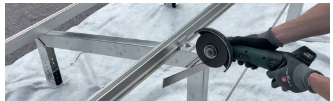
Figure 30: Cutting off the overhang from the wind bracing.
