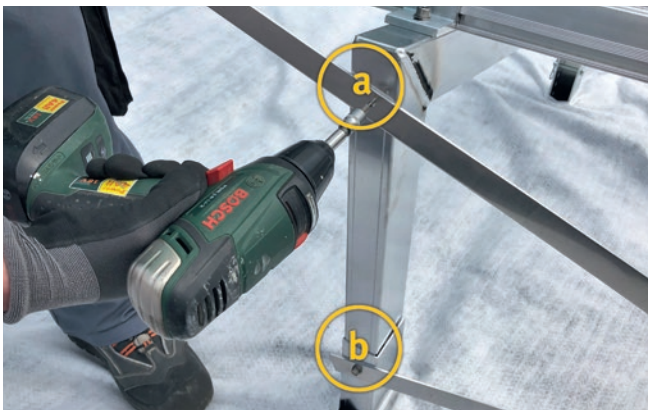
Figure 29: Position of drilled holes
