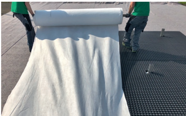
Figure 10: Rolling out the Filter Fleece.
