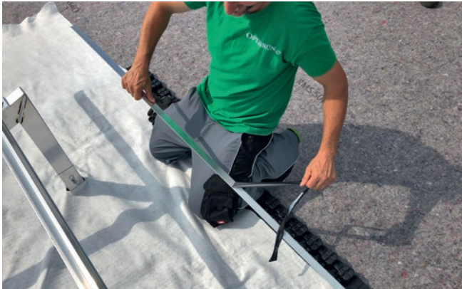
Figure 27: Removing the protective film from the wind bracing.
